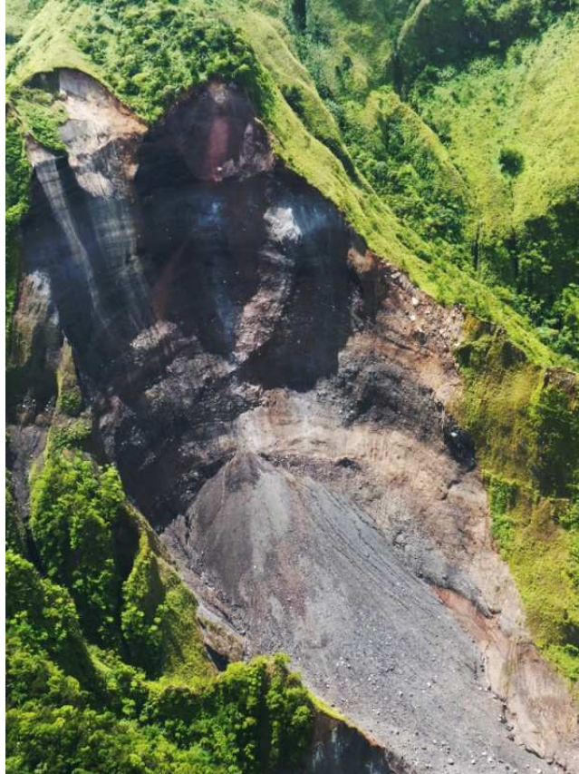
FIGURE 6.22. Collapse of the Piton Marcel in Martinique, France.
