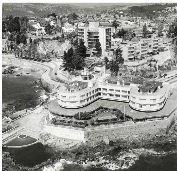
Fig. 51 Vista aérea Hotel Miramar, 1950. Tomada de: https://i.pinimg.com/originals/6b/b9/34/6bb934a35f32ccc83b1366213cd7c86e.jpg
