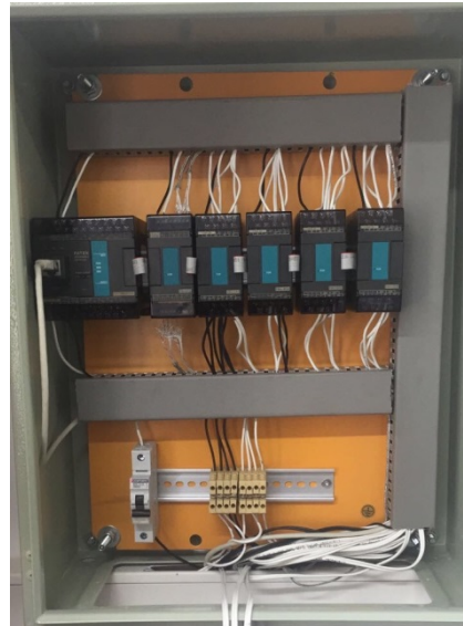
Figure 16: PLC board (left) and the units required for the communication of all the instruments (order corresponding to Table 3).
