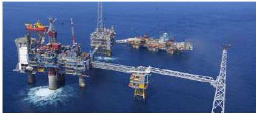
Figure 8 Project Sleipner facilities 2014, Stavanger, Norway. Global CCS institute. (Global CCS institute, 2018)
