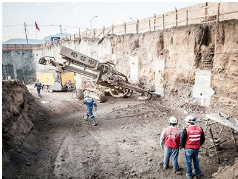
Figure 3 Anchored piles from the excavation of Los Trapenses Mall, Terratest.
